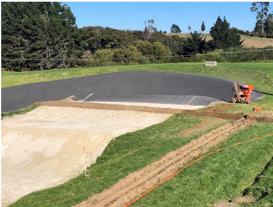
Trenching across track to reach corner exit.
