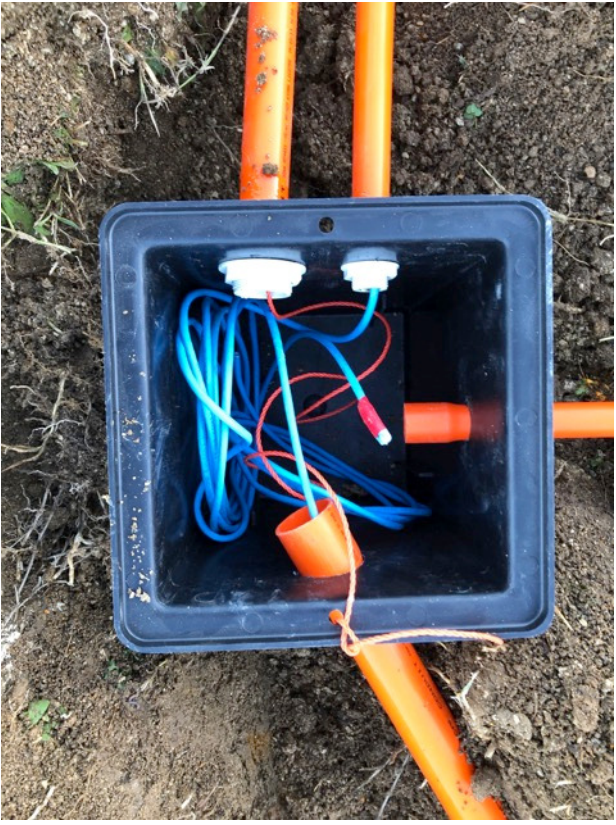
Access pit – Collecting 1 x 32mm, 2 x 25 with 40mm back to points hut/decoders. Total of 5 loops and 2 x Network
