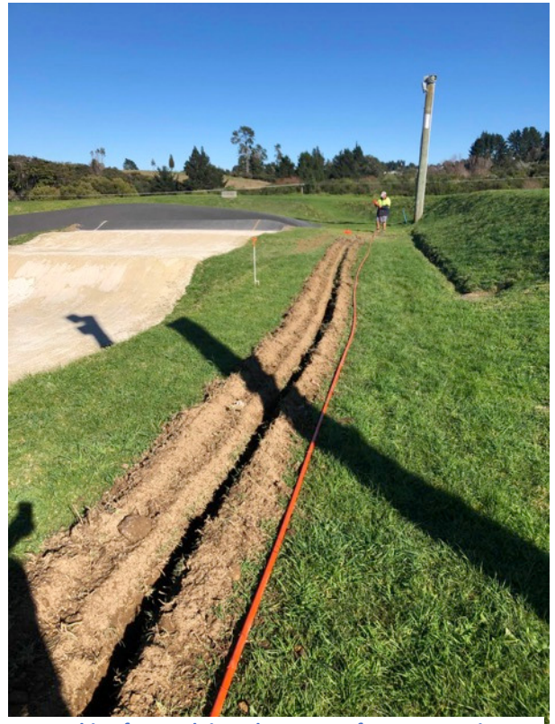
Trenching for conduit and coax runs from access pits to loop locations around the track.
