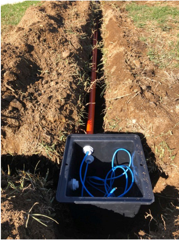
Access pit – Collecting two loops then back to decoder using 3 x 25mm conduit
