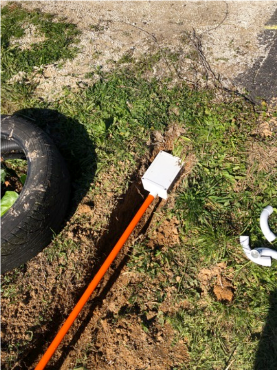
Enclosure beside the track for loop termination to coax.
